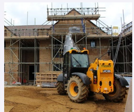
Solar panels go on to Cullum House
