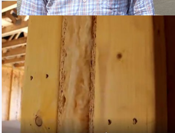
Sheep wool forms the insulation between two flats in Hook Norton
